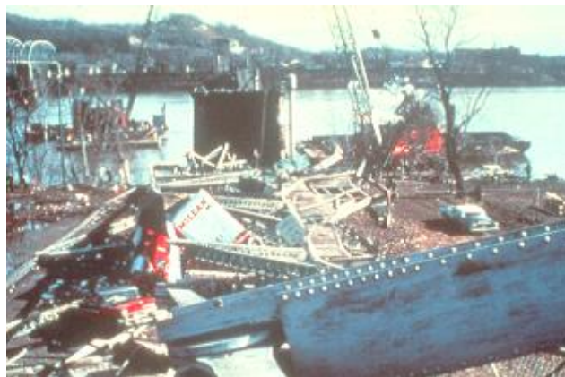
Figura 2-6 - Colapso da Silver Bridge, 1967 (Bridge Inspector's Reference Manual, 2006)
