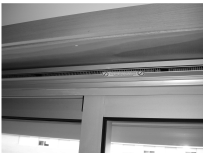
Figure 7. Ventilation grids on window frames.
