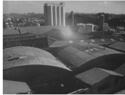
Figure 2. Aspect of the local before the intervention.
