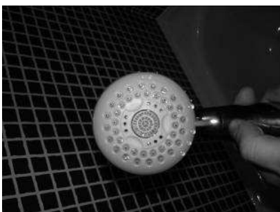
Figure 5. Low flow showers.
