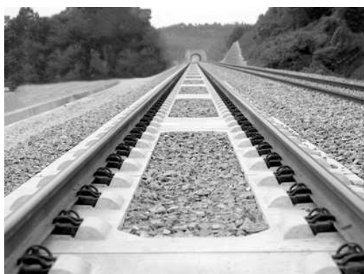
Figure 1.8: Slab-track
