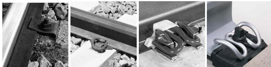
Figure 1.5: a) Nabla clip, b) Pandrol clip, c) Pandrol fastclip, and d) Vossloh clip
