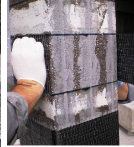
3. application of the epoxy resin to bond CFRP strips
