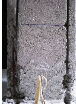
1. The too damaged concrete cover was removed
