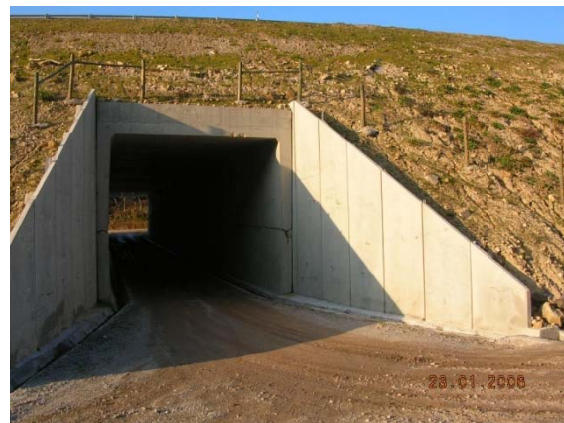
Fig. 1 – Examples of application of box-culvert.
