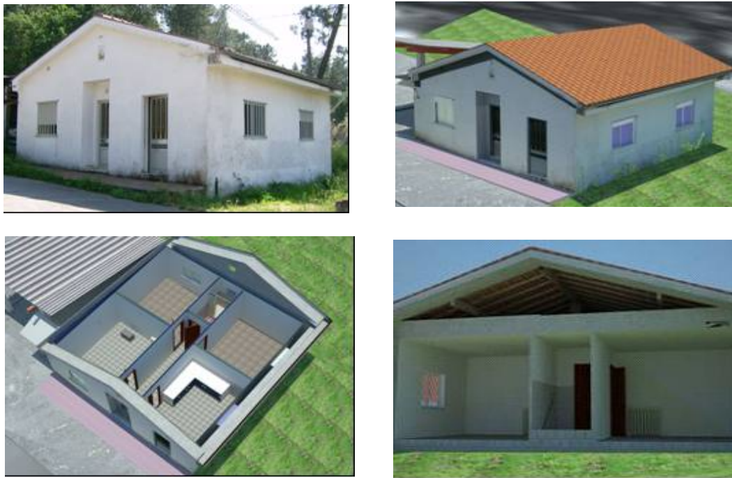
Figure 4. Case study with retrofit needs: a) photograph; b) exterior 3D model; c) interior 3D model; d) 3D model cross-section;
