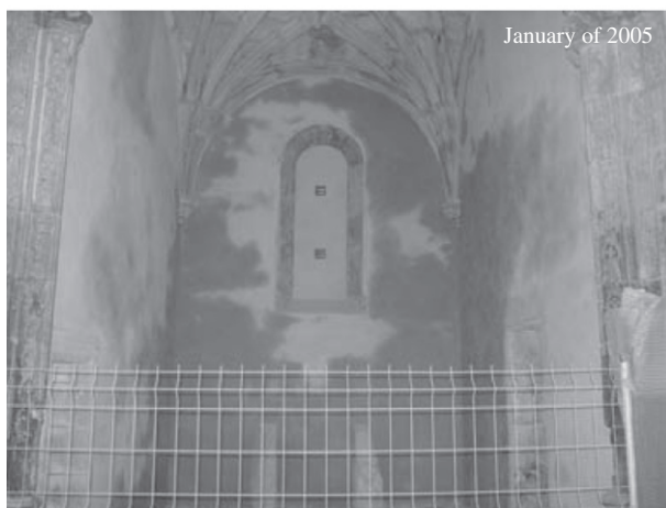
Fig. 1. Drying of a lime-based rendering inside a church in Portugal [4].
