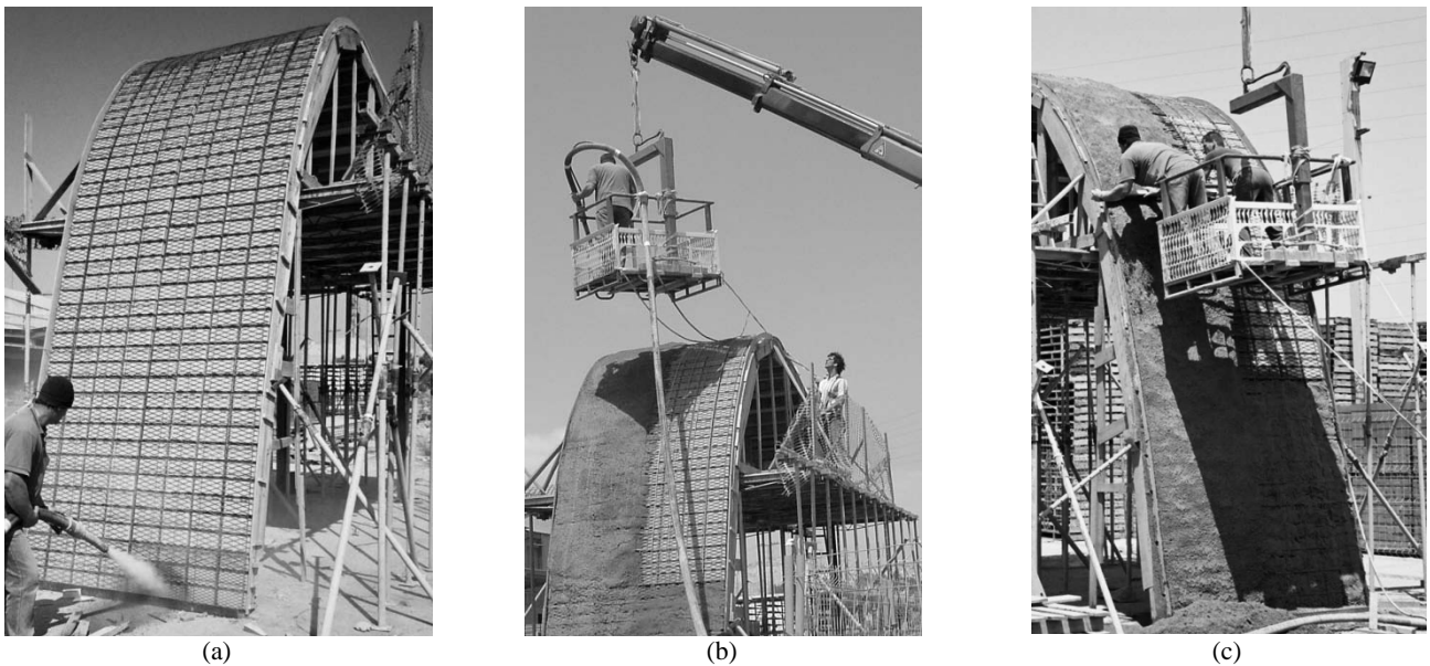
Figure 16. Third solution for concreting (High Pressure). Sprayed mortar
