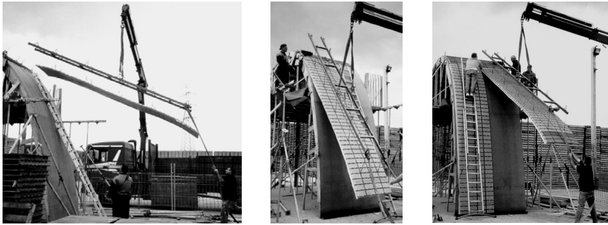
Figure 12. Placement of sheets on the falsework
