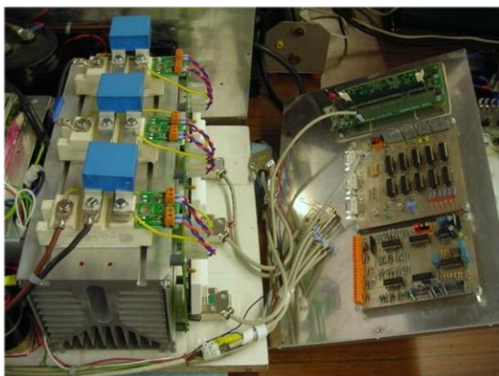
Figure 6: Developed prototype of the smart bidirectional batteries charger.
