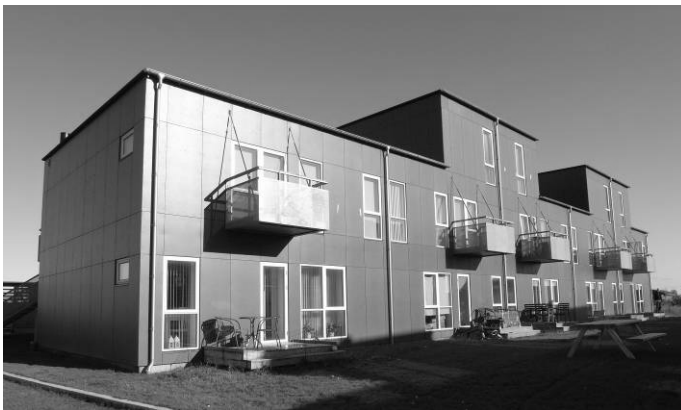
Figure 2. Photo of the KAB-ultralow-energy housing project.
