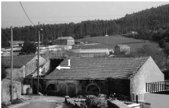
Figure 1. Watermill building's condition in 2000
