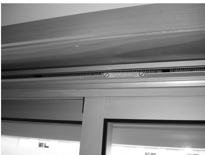
Figure 7. Ventilation grids on window frames.
