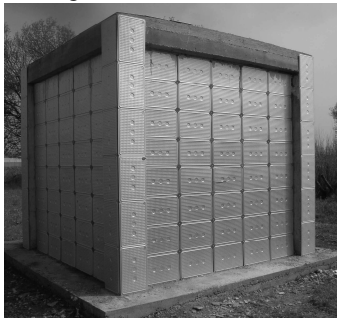
Figure 4. Brick cubicle with RT-27 and polyurethane.
