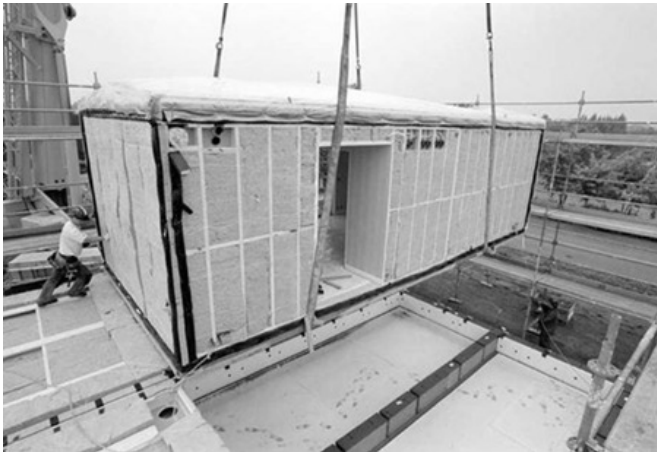
Figure 1. IKEAS' Boklok house installation.
