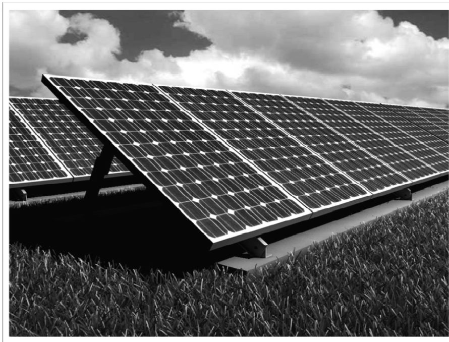
Figure 11. Rail mounted thick-film crystalline PV panels on rail mounted system at the Turkey Lake Service Plaza
