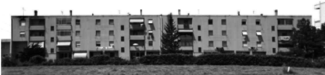
Fig.1 The existing building
