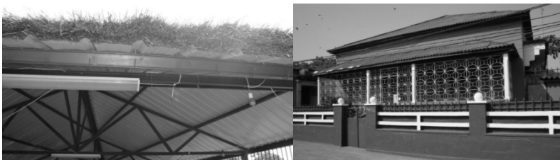
Figure 3. Double roof system, with zinc foil under a straw-covered roof. Colonial dwelling.
