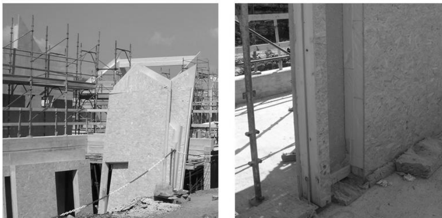
Figure 7. Prefabricate external wall panels.
