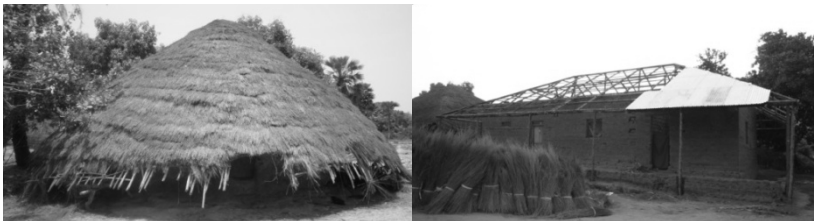
Figure 2. Vernacular architecture (left). Replacing straw roof with zinc (right).
