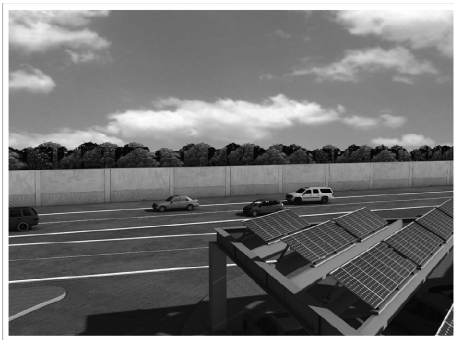
Figure 13. Crystalline engineered structure mounted on rail system in open areas of the Turkey Lake Service Plaza
