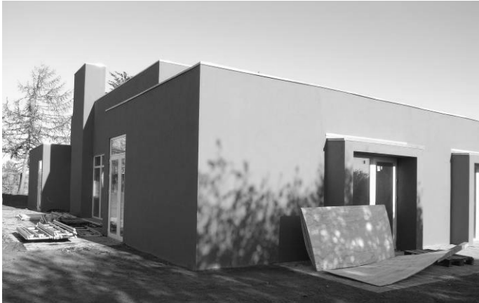
Figure 4. Photo of the centre for senior citizens – under construction.
