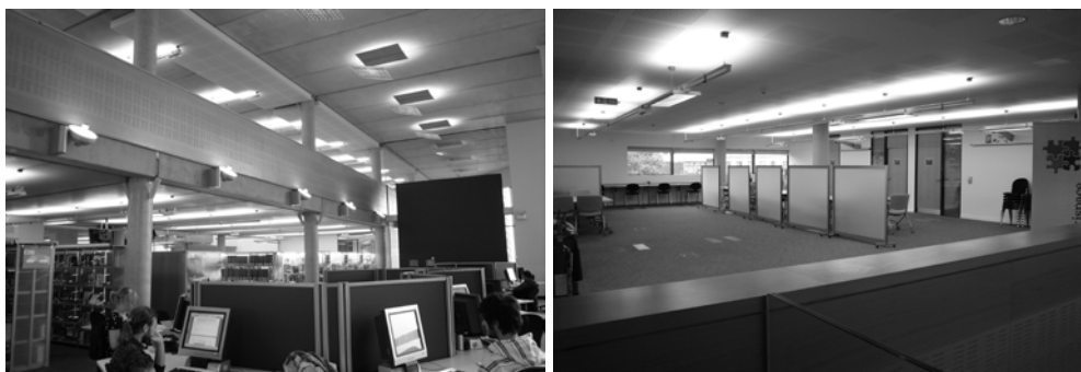
Figure 10: The uplighter used in double height floor area (left); dark grey and deep textured surfaces, which resulted in the 'hot spot' and the dark appearance of ceiling (right)
