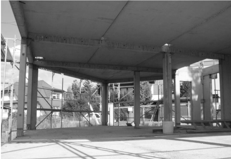
Figure 6 Light precast RC frame structure
