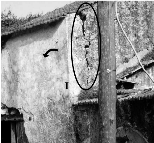
Figure 9. Vertical crack, 2007
