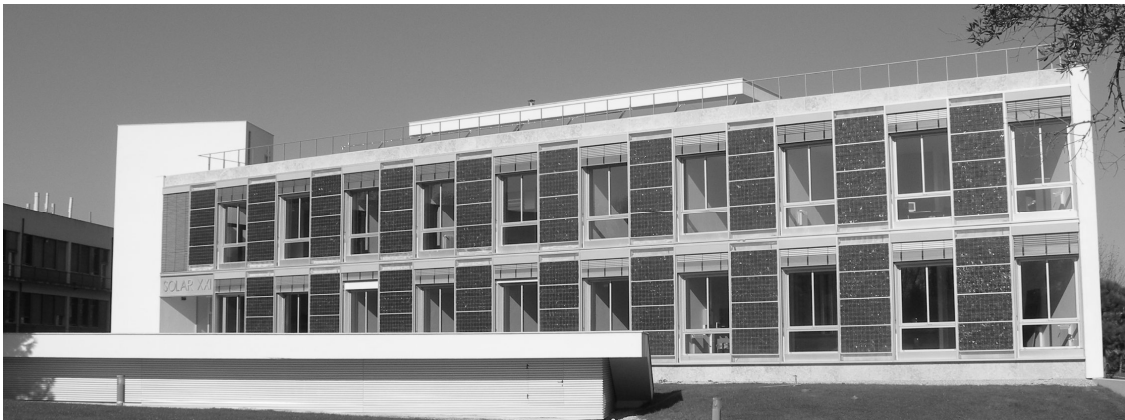
Figure 1. Direct gain and PV panels in south façade of Solar XXI building.
