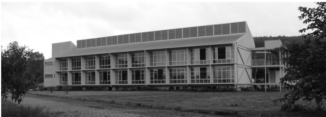
Figure 1 – South Facade with glazing and protected plans
