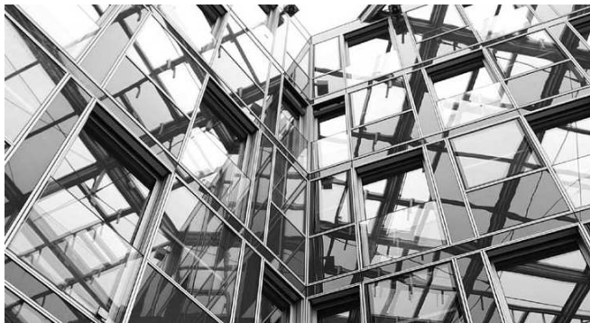
Figure 2. Capricorn Facade. Reference: Schneider Electric. Capricorn Haus, 2009.
