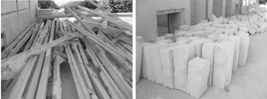
Figure 3. Dismantling and waste classification: RC roof elements and wall masonry elements.
