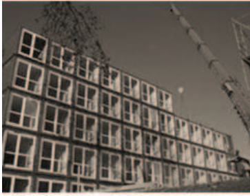
Figure 1. Left: City of modular steel containers, Keetwonen
