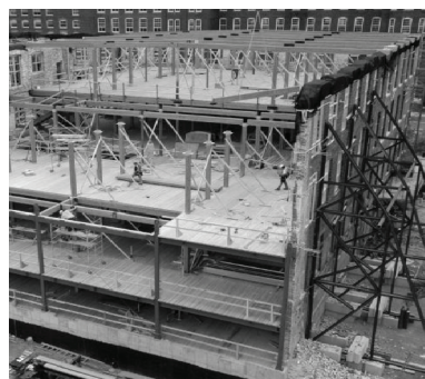
Figure 6. System of posts and beams
