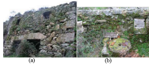
Figure 2. Construction 39 (Mill): (a) North elevation; (b) millstone. Credits: Authors.
