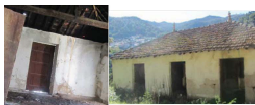
Figure 5. Construction 38 (house) – roof with tile. Credits: Authors.
