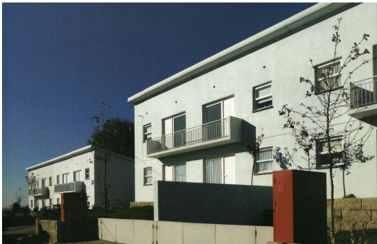
Fig. 2 Building front view, after renovation
