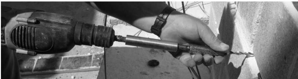
Figure 6: Insertion of Heli ® -needle with the hammerhead prototype.
