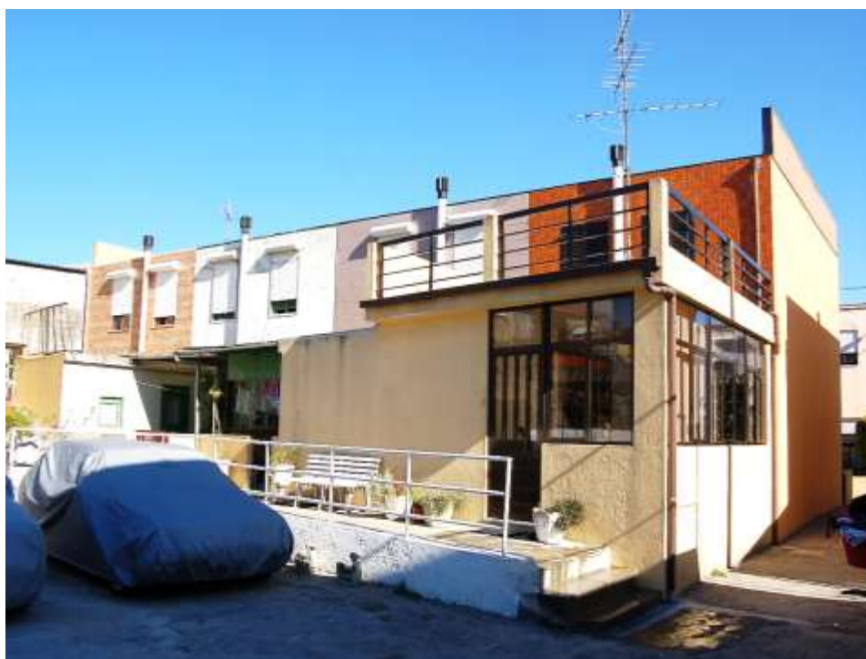
Figure 3. SAAL Porto, dwellers' alterations in Maceda housing (Alcino Soutinho, 1975-76): addition of new volume (occupying areas intended for external private spaces) and changes in the colour and material on the exterior walls, which were initially painted in white (photo by the author, Jan. 2006).
