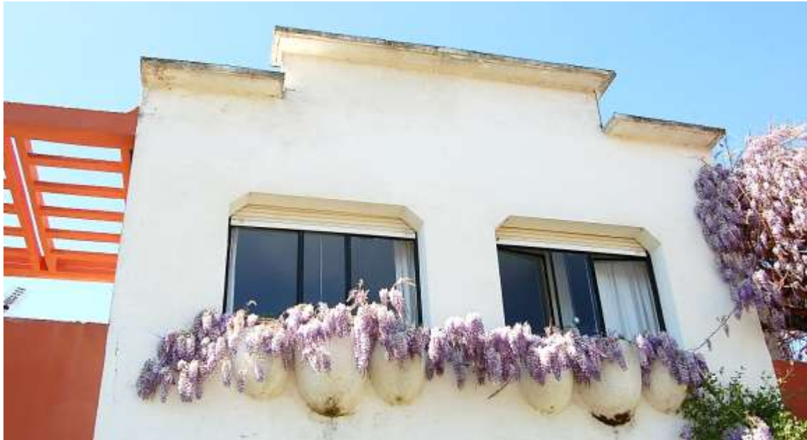
Figure 2. Closer view on the dwellers' alterations on the 'type Quinconce ' house shown in figure 1 (photo by the author, June 2007).
