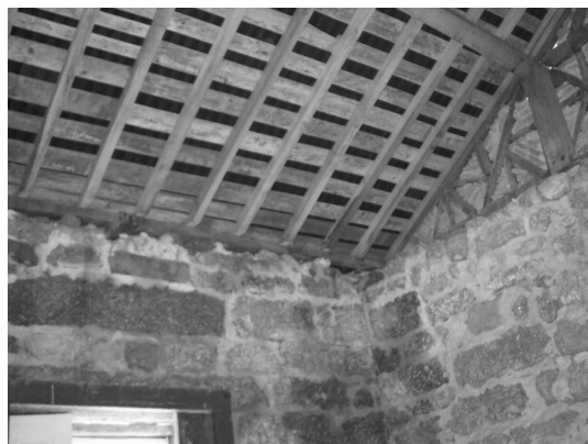
Fig. 2 - Inner view of a building with stone walls and timber roof.
