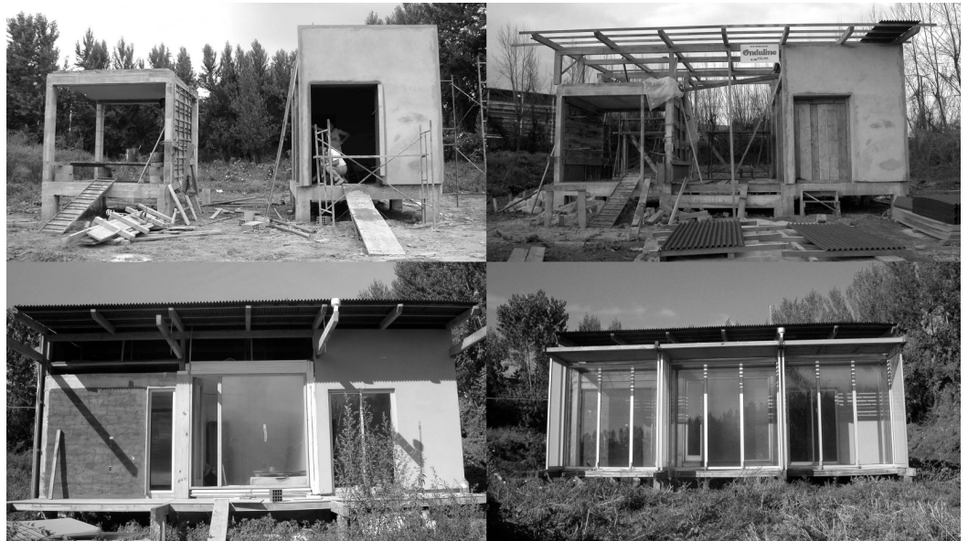
Fig. 10 - Exterior views of the building test cells construction works.
