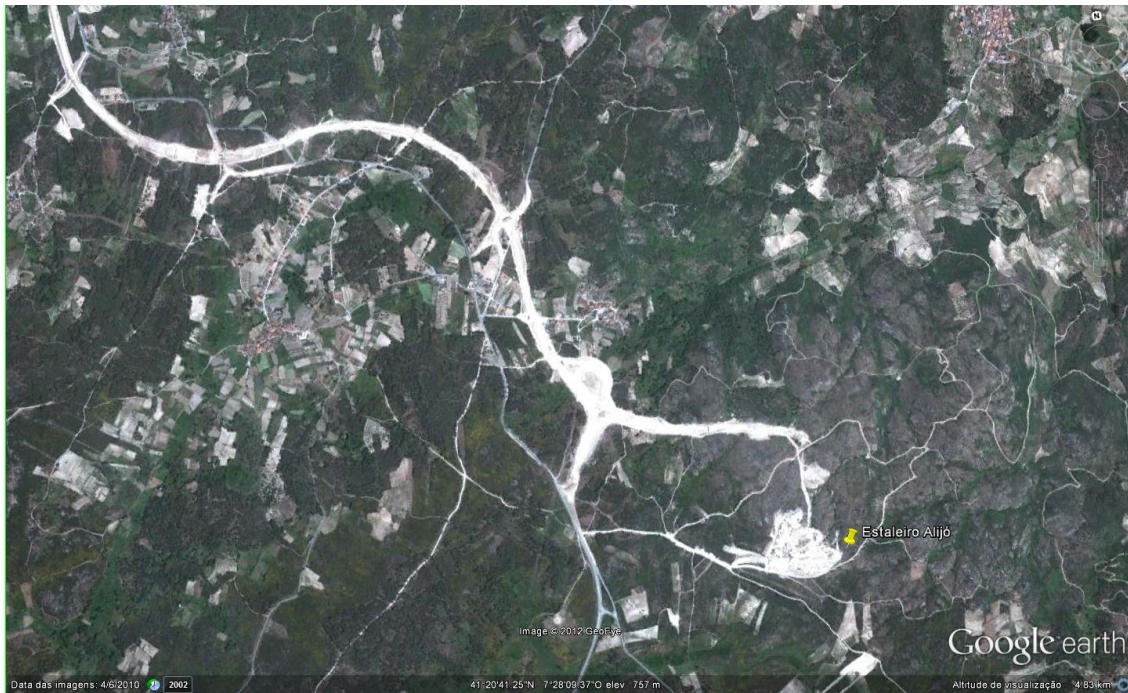
Figure 5.3 Aerial image of construction site ( Google Earth )
