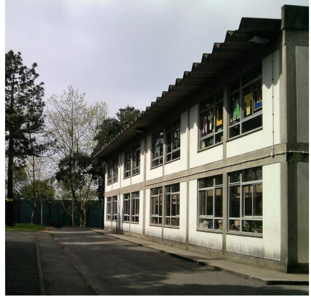
Figure 3. View of the East façade of the school, relative to the classroom area
