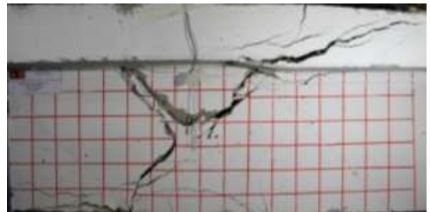
f) Final crack pattern of the NSM-3L45 beam
