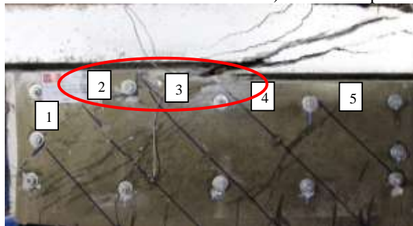
f) Final crack pattern of the SP-5L45-B beam
