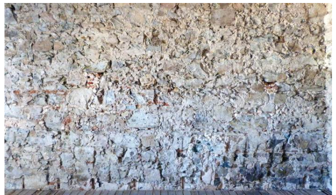
Figure 9. Stone masonry morphology.
