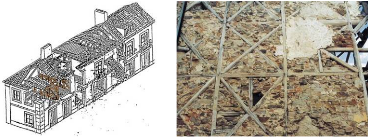
Figure 2. (left) Use of frontal walls in two-story buildings in Vila Real de Santo António (Mascarenhas 1996); (right) Frontal wall in Vila Real de Santo António (Figueiras 1999).
