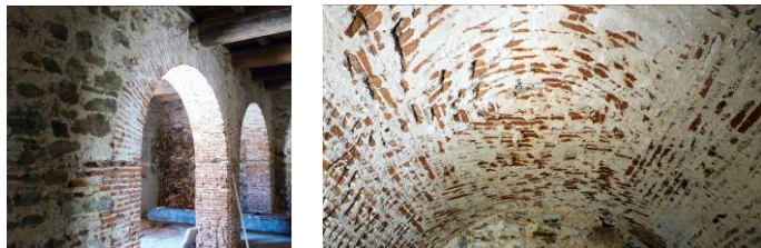
Figure 6. (left) Brick masonry arcades (right) brick masonry barrel vault.
