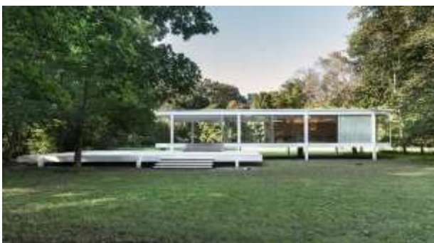
Figura 3 - Farnsworth House, 1951. Mies van der Rohe
