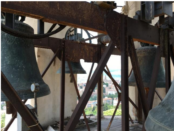
Figure 3-7 Bells supported by the metal structure
