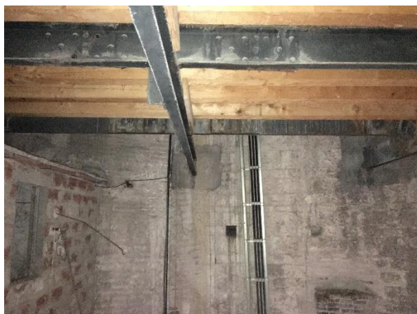
Figure 4-4 Beams embedded in the shaft
