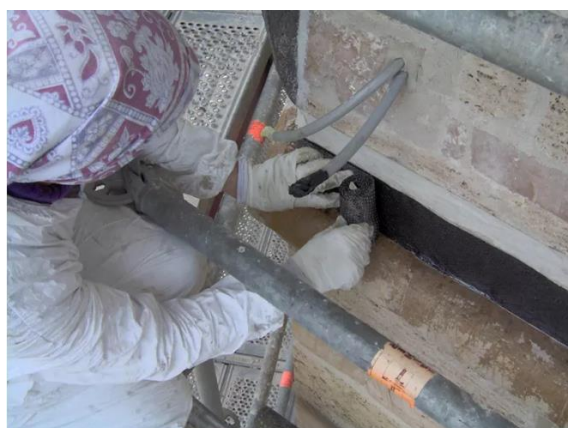
Figure 3-9 Application of FRP materials during the last restauration works [30]
