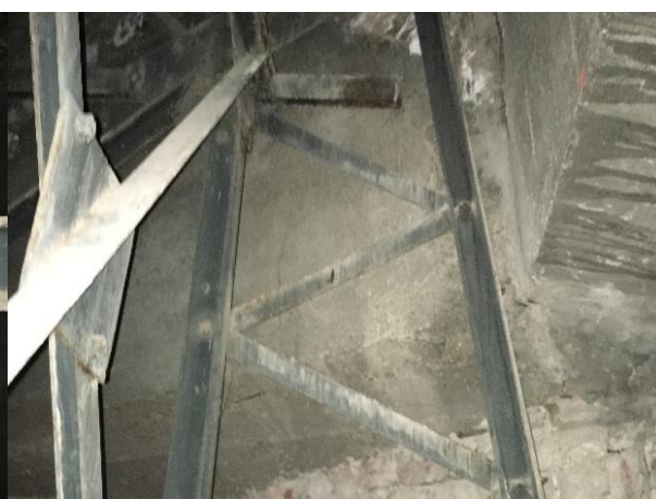
Figure 4-9 Example of oblique lateral support
