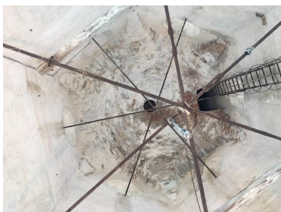
Figure 3-5 Tie rods in the belfry
