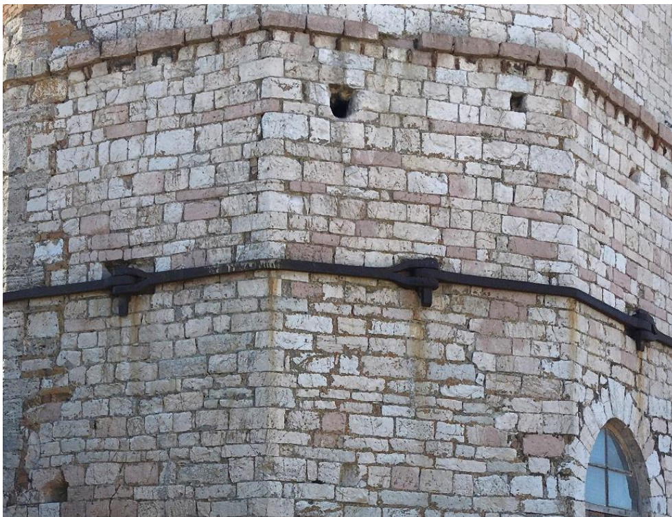
Figure 4-2 Exterior masonry of the shaft
