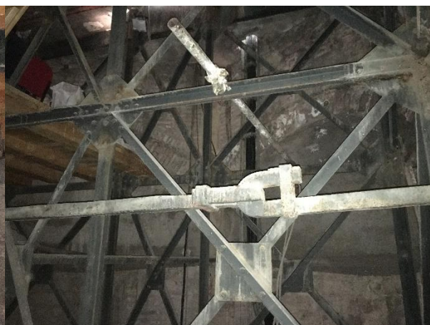
Figure 4-5 First and second level of the metal structure
