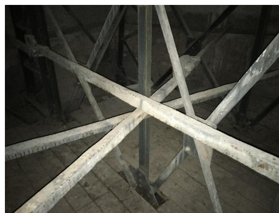
Figure 3-4 Tie rods in the shaft
