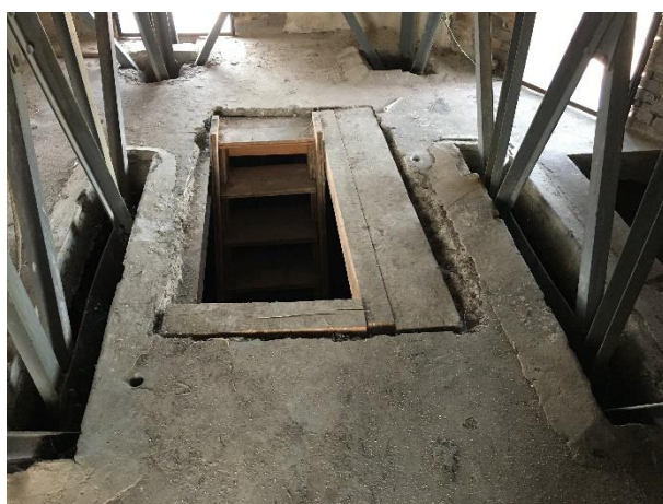
Figure 4-6 Concrete floor crossed by the metal structure
