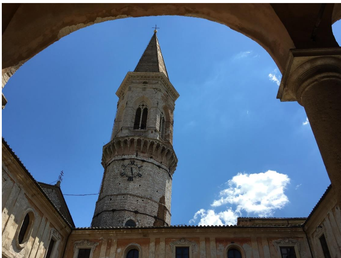
Figure 3-1 North-West side of the bell tower
