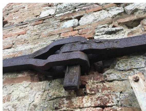
Figure 3-6 Detail of metal confinement
