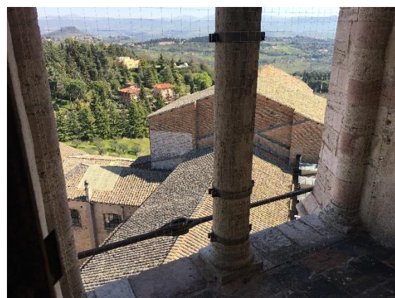
Figure 3-10 Confining elements in double-arched windows
