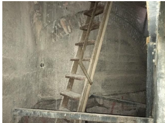
Figure 3-8 Concrete elements supporting the lateral arches of the demolished vault
