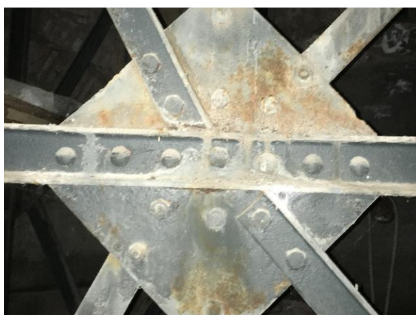
Figure 4-8 Example of connection between profiles
