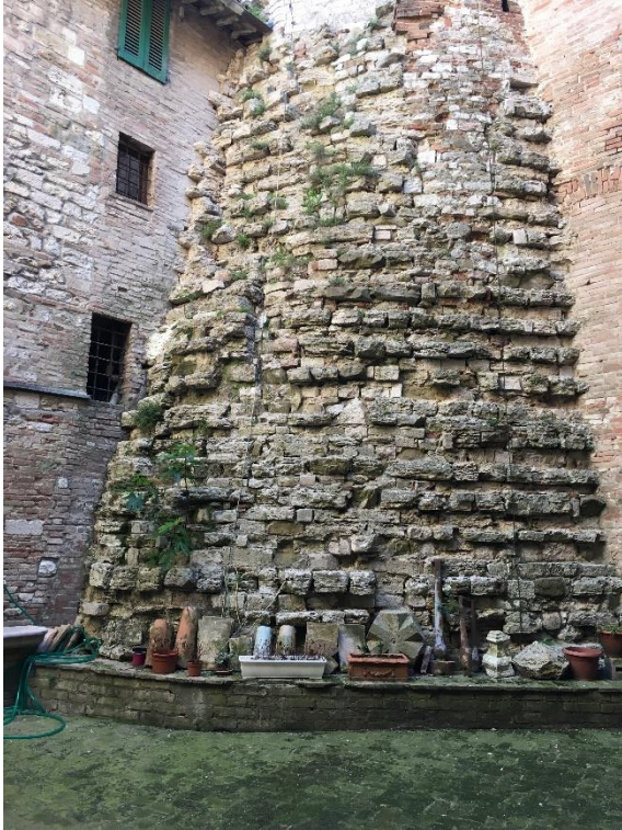
Figure 3-13 Basement of the tower
