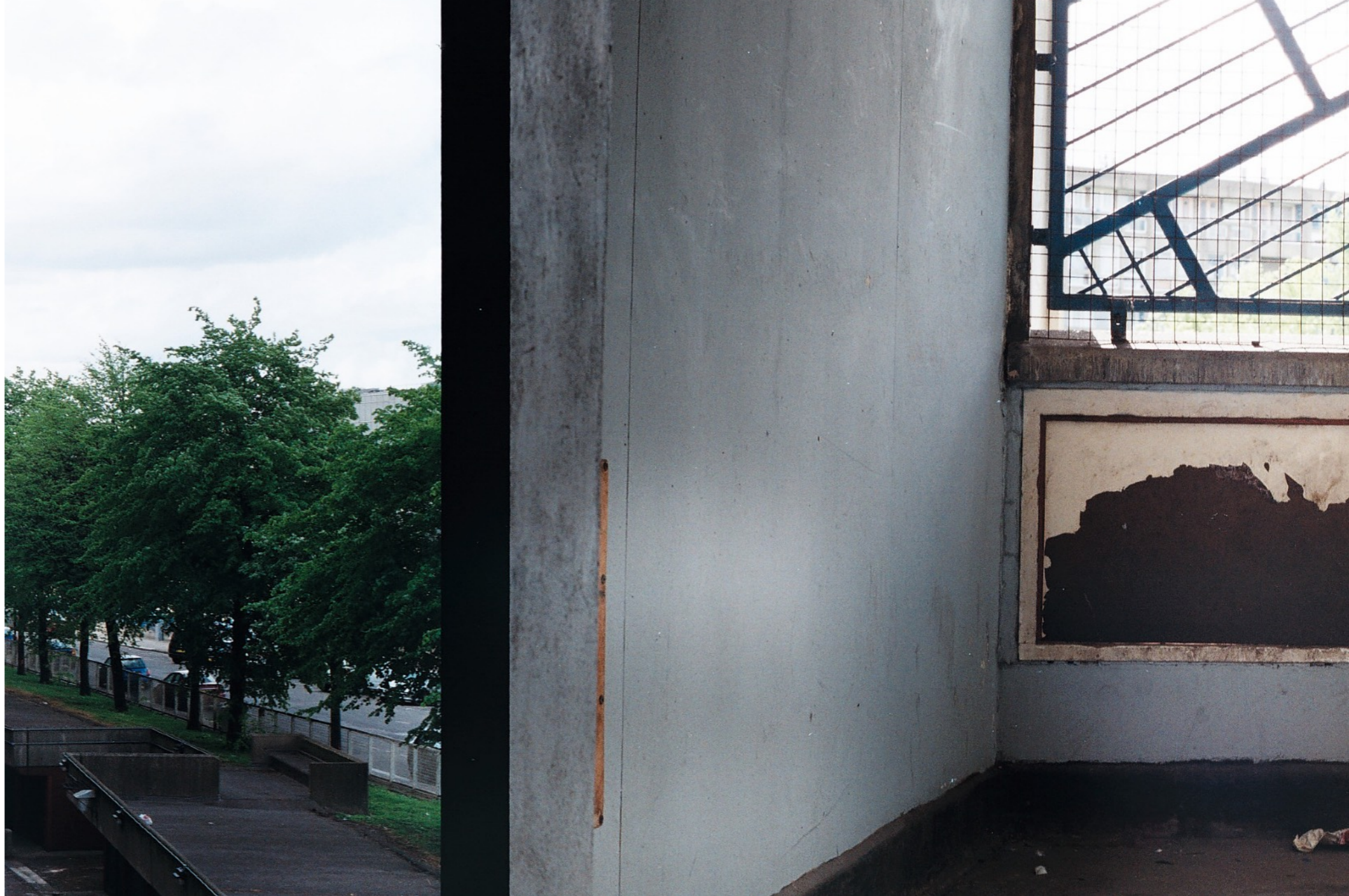
Vertical accesses in Robin Hood Gardens. Photo by Fernando Ferreira, 2014 ©
