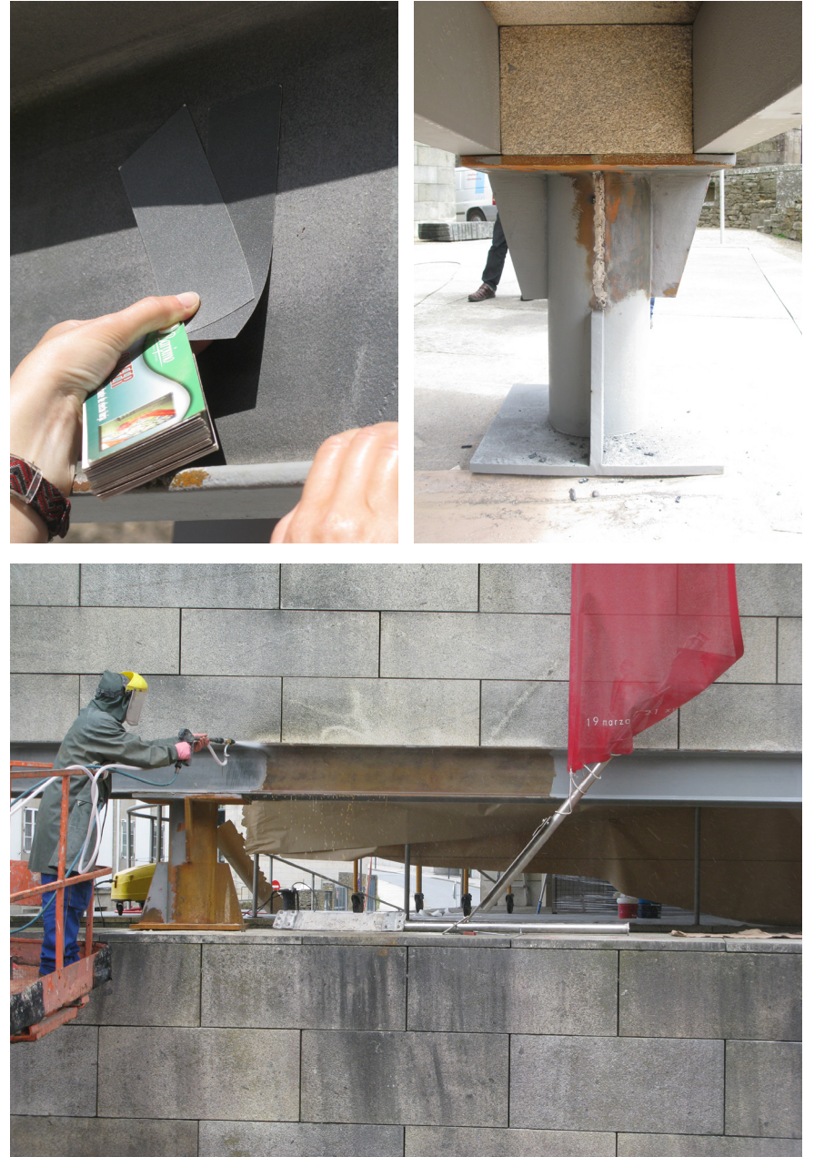
Fig. A12 and A13 Process of restoration of the exterior surfaces.
