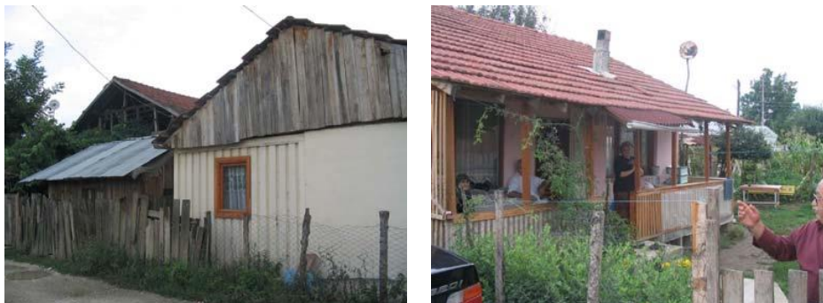
Fig. 38: in Turkey, A family of four has modified, over three years, a shipping container donated to them as a temporary house into a permanent house with the addition of extra rooms and traditional Turkish sofa (veranda). Side view of the house (left) and front view of the house and the family (right). (Johnson 2008, 331).
