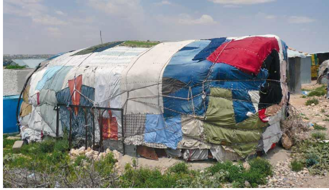
Fig. 8: Self-built shelters in Somalia, based on the traditional 'Buul'. In cities, they are built using recycled fabric, cardboard and tin cans. Photo by: Joseph Ashmore.
