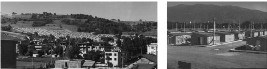
Fig. 33: Views of the temporary housing settlement built in the outskirts of the cities of Adapazari and Izmit, Turkey. Source: (Johnson, Lizarralde, and Davidson 2006, 372).
