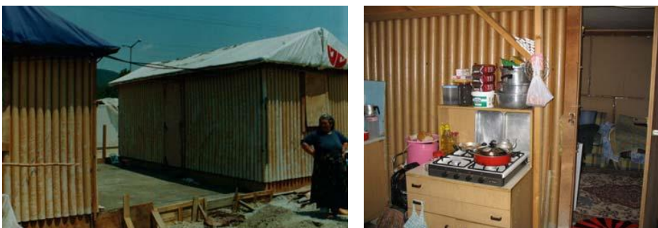
Fig. 39: In Turkey, A lady consolidates two paper temporary houses into a three-room dwelling with the addition of a kitchen and bathroom in the middle. View of the two units and the concrete foundations for the kitchen in 2000 (left) and inside view of kitchen built between to the two paper houses in 2004 (right). (Johnson 2008, 331).
