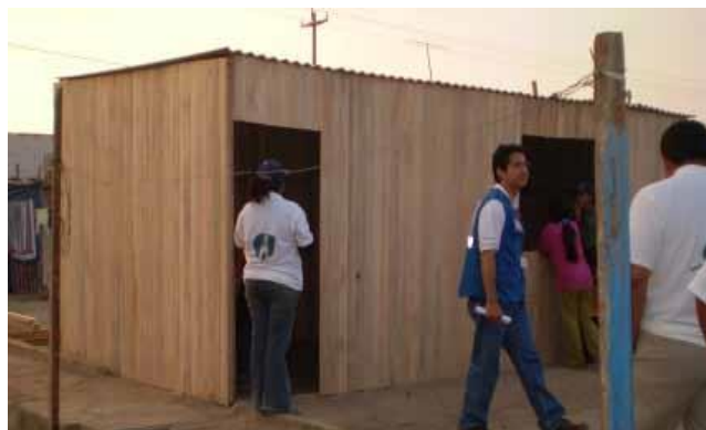
Fig. 25: Timber Frame following earthquake in Peru 2007. Source: (IFRC 2011, 45).
