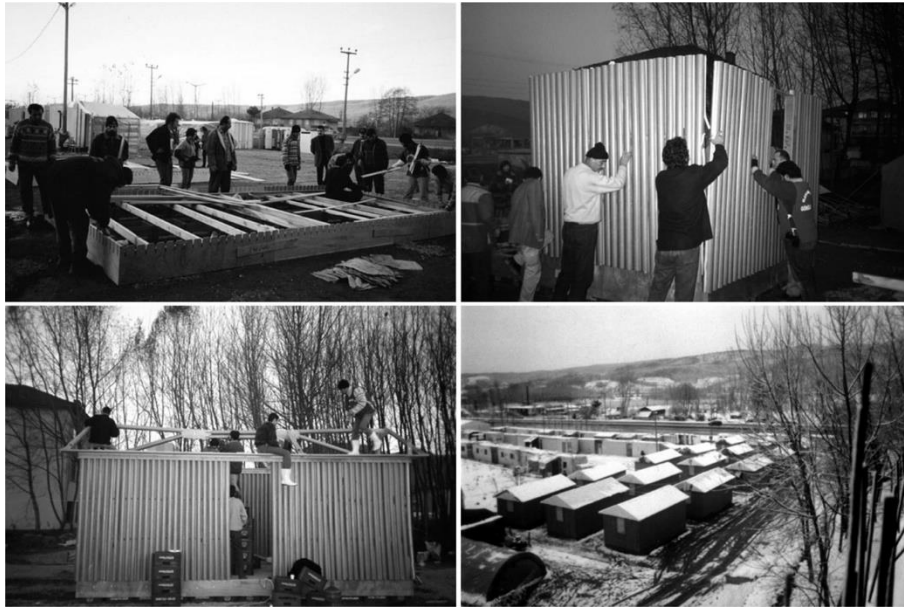
Fig. 24: Kit solutions: assembly process by local community and cluster of the Paper Log Houses designed by Shigeru Ban. Source: https://archnet.org .
