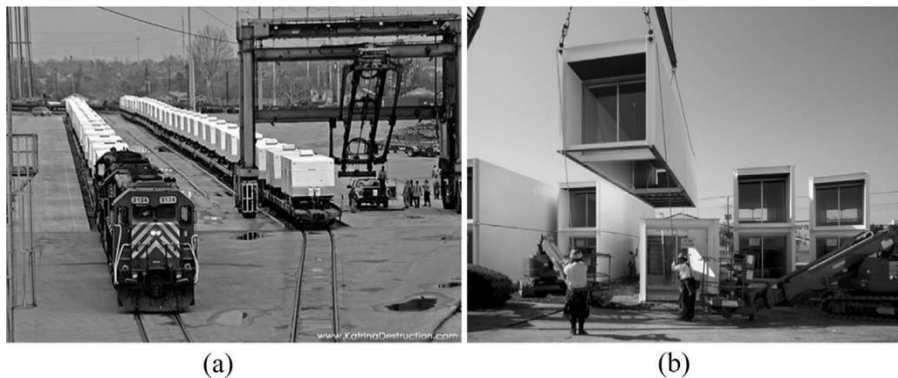
Fig. 23: Ready-made units: (a) temporary housing units ready to be transported (source: www.katrinadestruction.com ), and (b) local assembly of units. Source: http://exc.ysmr.com .
