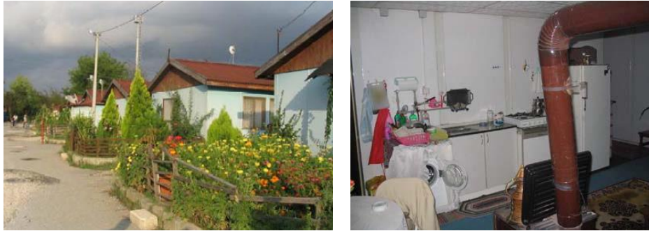
Fig. 36: In Turkey, Kiremit Ocağı settlement near Düzce town centre has become rental housing, most residents have planted gardens (left); in the UMCOR settlement, a family that rents two connected units, has taken down the partition wall and now occupies 50m 2 . Source: (Johnson2008, 330).
