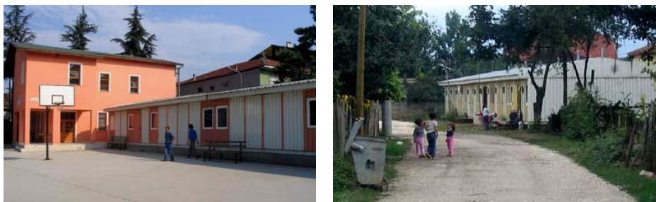
Fig. 37: In Turkey, an eight-unit building that is part of the UMCOR temporary housing settlement (left); units reused as classrooms at a school (right) after being dismantled, moved across town and reassembled. Source: (Johnson 2008, 330).
