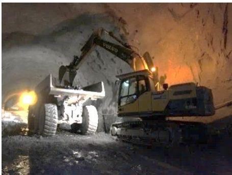
Fig.123-Carga de dumper com escombros[31]
