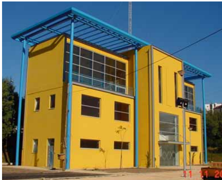
Fig. 1 - Front and lateral view of the building
