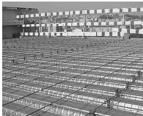
Figure 7. General view of the MBT floor construction
