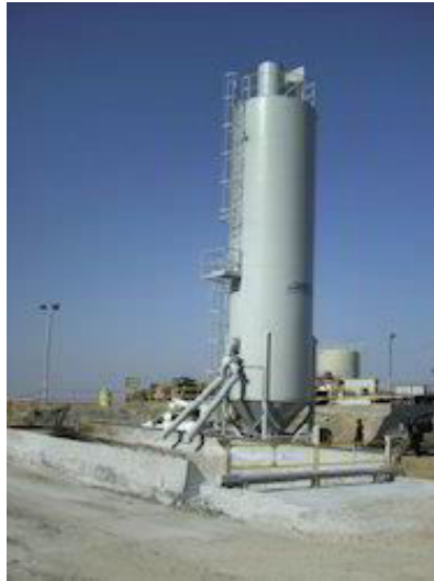
Figure 7 - Cement Storage Silo.
