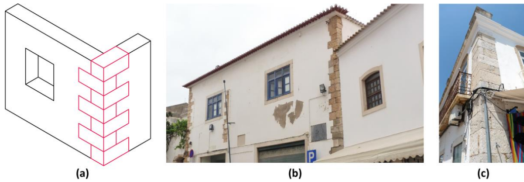
Figure 2.9: (a) Traditional ashlar stone masonry quoin; (b) stone masonry quoin in Lagos, Portugal; and (c) ashlar stone masonry quoin in Vila Real de Santo António, Portugal
