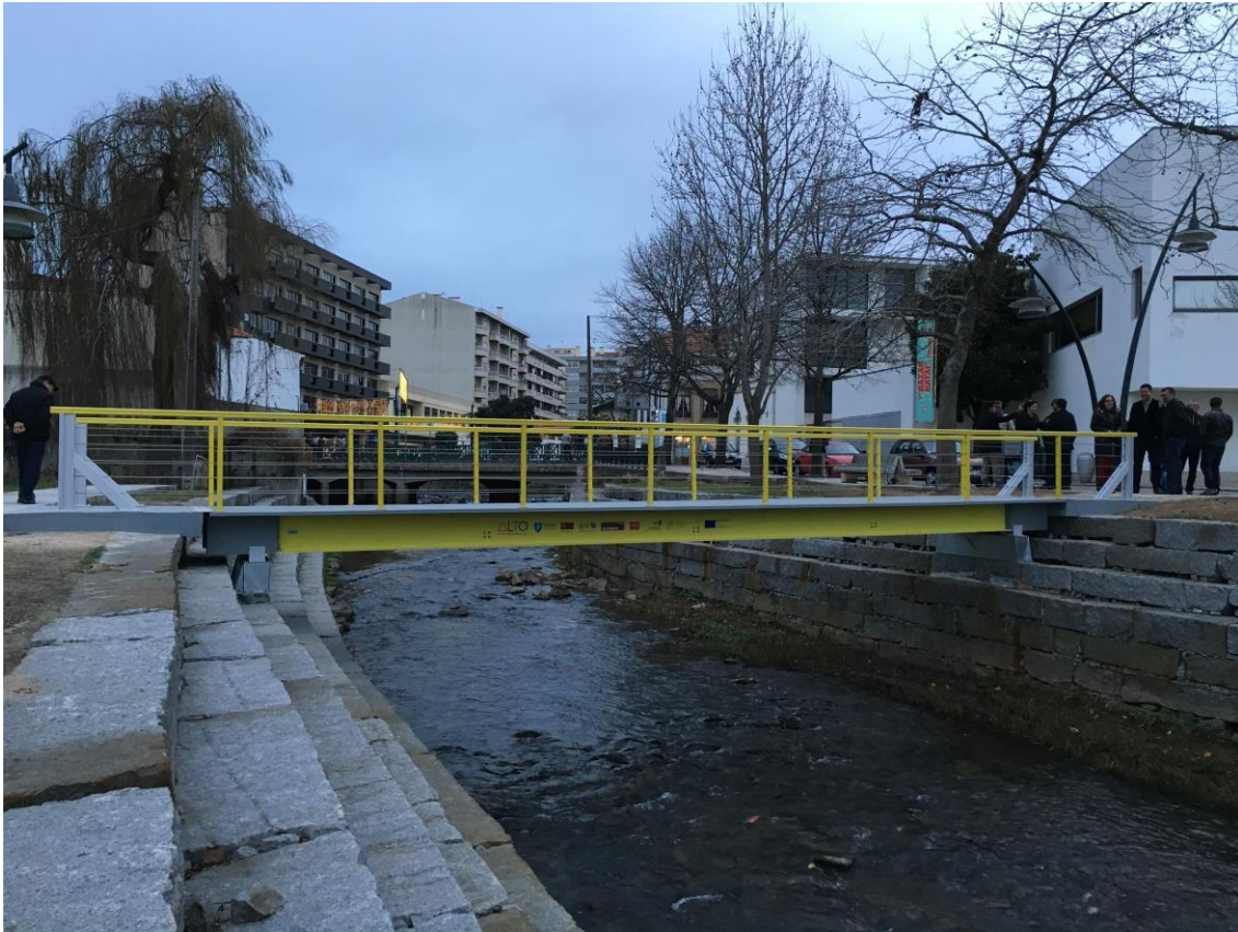
Figure 22 – São Silvestre Bridge (Pontalumis project), Ovar, Portugal.
