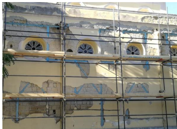
Figure 2.8 Anti-rust protection of the iron frames of the external walls
