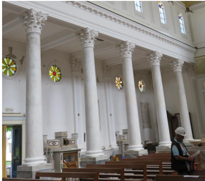
Figure 3.24 Unresolved node of the connection between the columns, the central nave second floor wall and the iron floor of the side aisle
