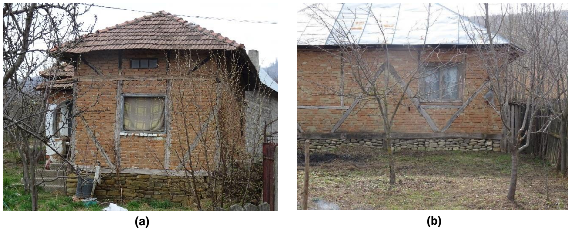
Figure 2.33 Timber frame geometry of building in Ocnești (a) and Vrancea (b), Romania (Dima and Dutu 2016).
