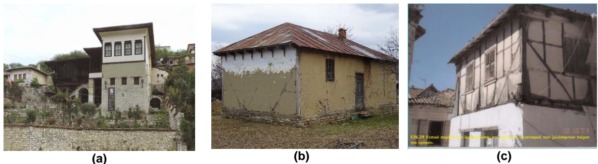
Figure 2.4 Non-engineered TFM systems: Albania (a); paianta , Romania (b); Greece (c) (Vintzileou et al. 2004).
