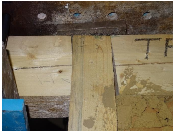
Figure 5.9 Negligible sliding between post and upper beam.
