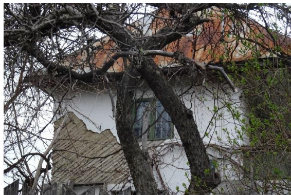
Figure 2.37 Building classified as Type 2 in Romania (Dutu et al. 2018b).
