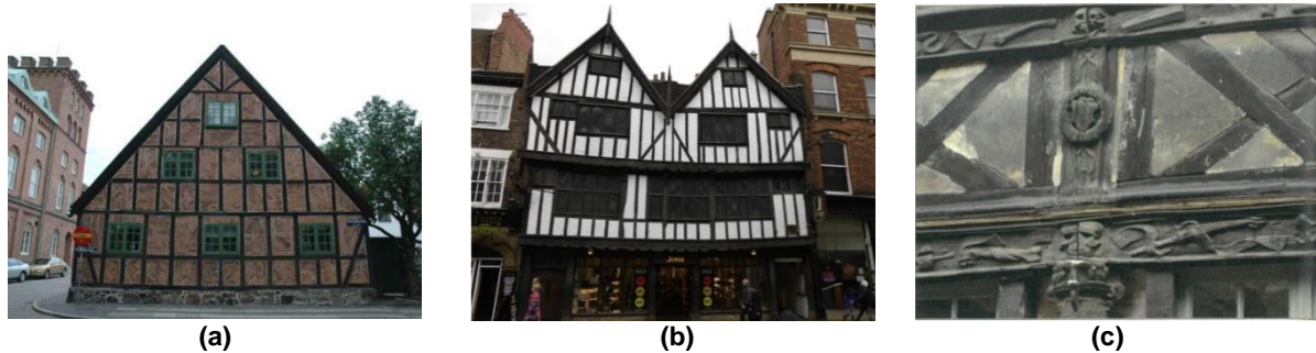
Figure 2.2 Non-engineered TFM systems: Sweden (a); half-timber, England (b); fachwerk, Germany (c) (Bianco 2010); (Copani 2007); (Lukic 2016).
