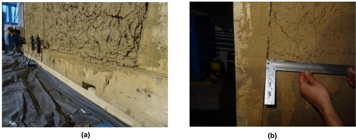
Figure 3.23 S3 damages: no out-of-plane mechanism (a), detachment of infill (b) (Dutu et al. 2018a).
