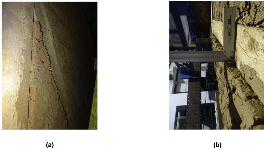
Figure 3.19 Out-of-plane of masonry infill S1 (a), S2 (b) (Dutu et al. 2018b).
