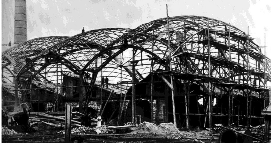
Figure 2.8- Pavilions built for the Nizhni Novgorod exposition (Edemskaya, 2014)
