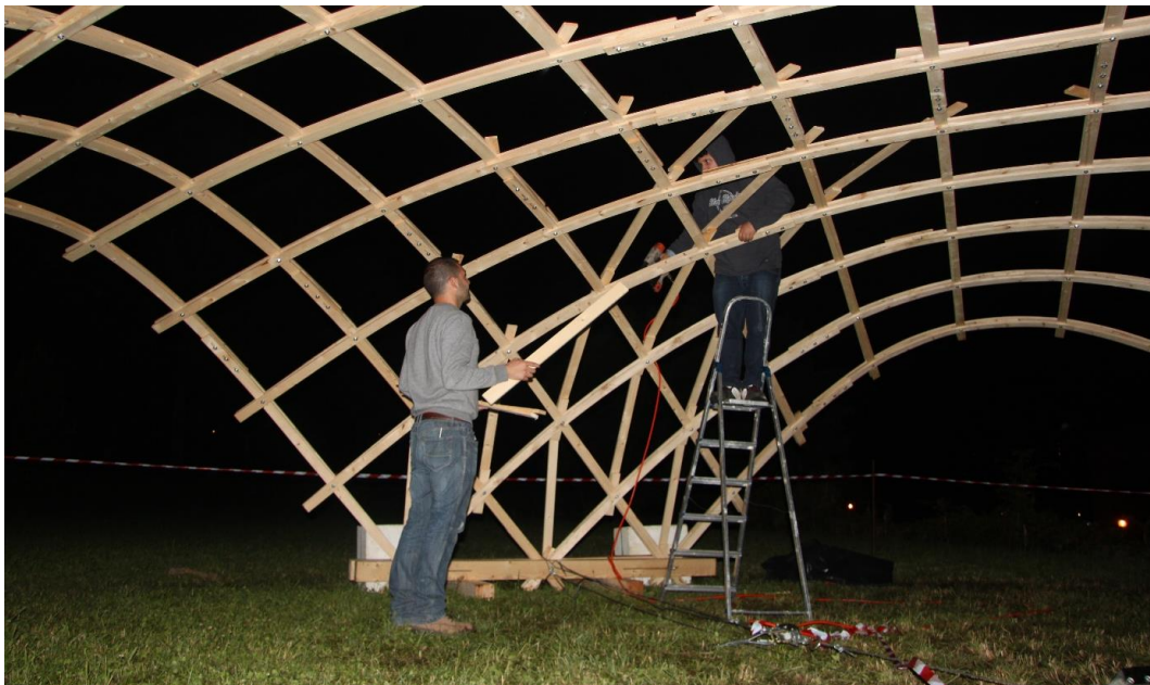
Figure 5.28- Application of locking with nail gun
