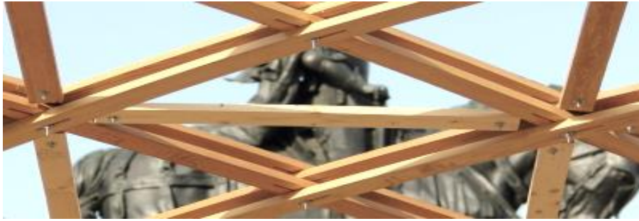
Figure 3.34- Locking detail of the ZA Pavilion (Richard Harris & Williams, 2014)
