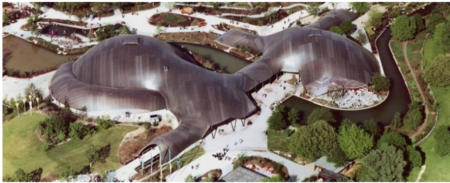
Figure 3.11- Manheim Multihalle (Verde & Truco, 2009)
