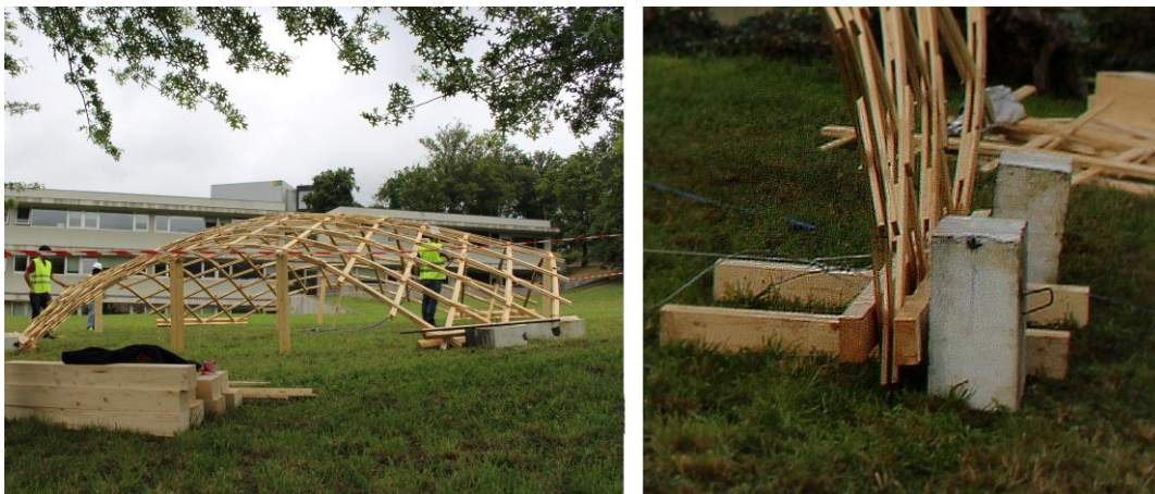
Figure 5.24 a, b- Gridshell Construction
