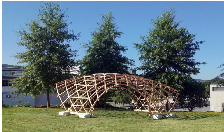
Figure 6.3-First elastic timber gridshell in Portugal
