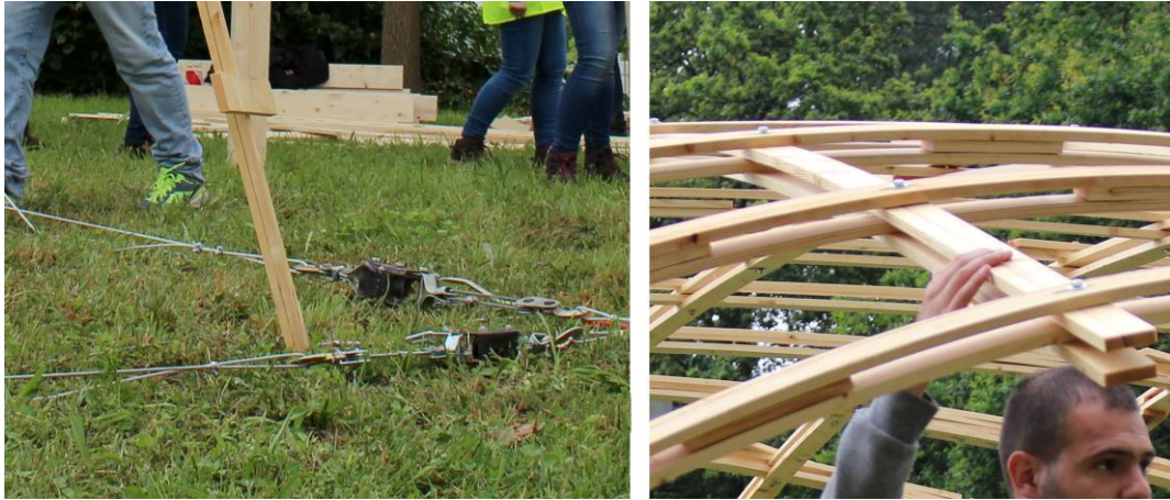
Figure 5.25 a, b- Gridshell Construction
