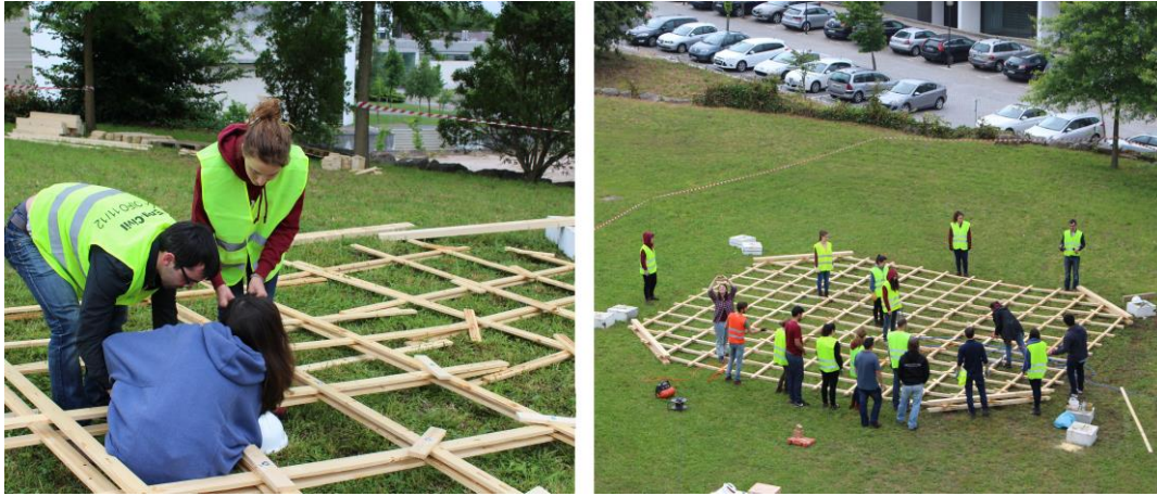
Figure 5.22 a, b- Gridshell Construction
