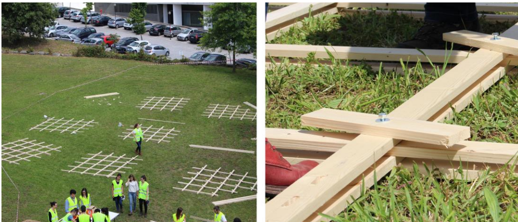
Figure 5.21 a, b- Gridshell Construction
