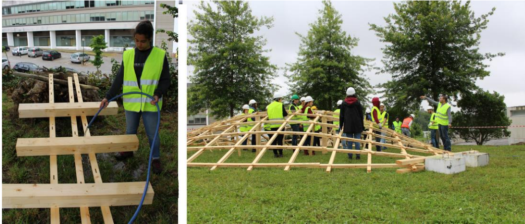
Figure 5.23 a, b- Gridshell Construction
