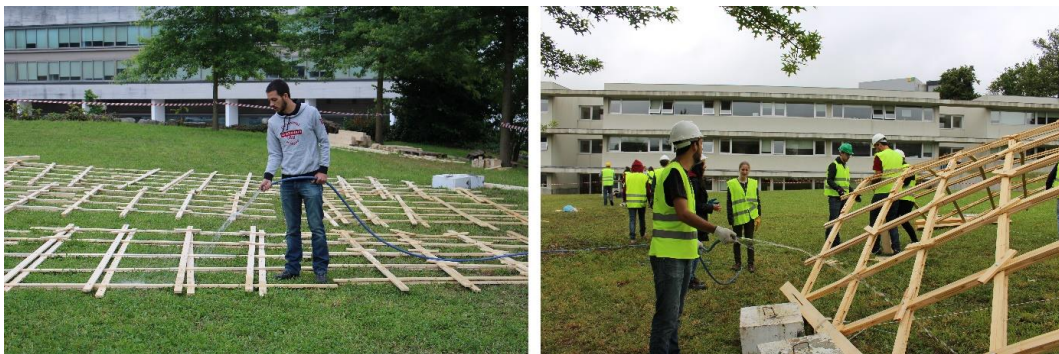
Figure 5.20- Moisturing of the timber elements
