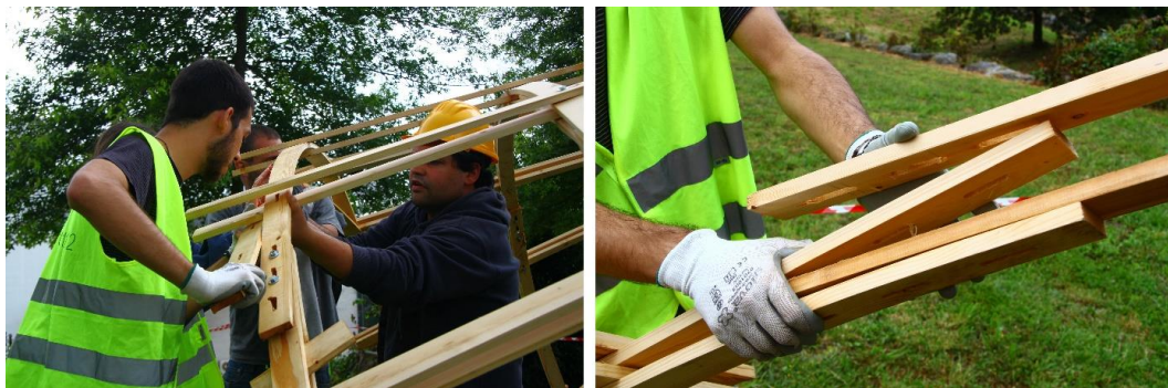
Figure 5.30- Replacement of damaged elements
