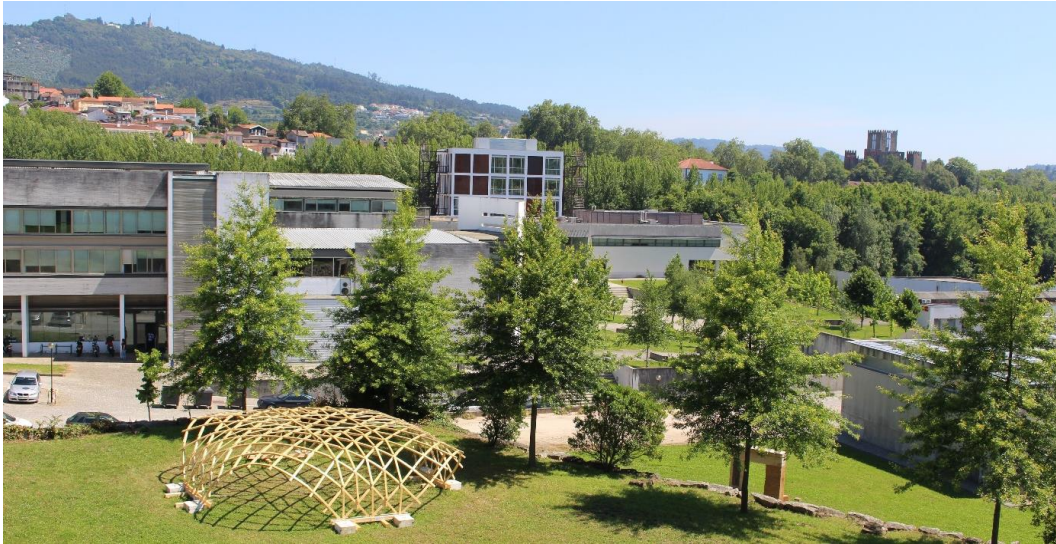
Figure 5.34- First structural mesh in wood, recorded in Portugal. Campus of Azurém, University of Minho, Guimarães
