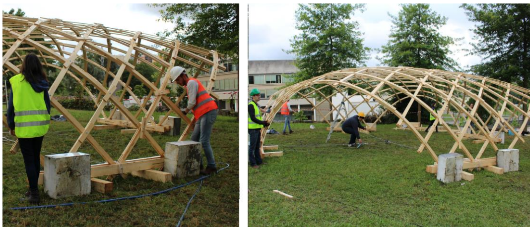
Figure 5.26 a, b- Gridshell Construction
