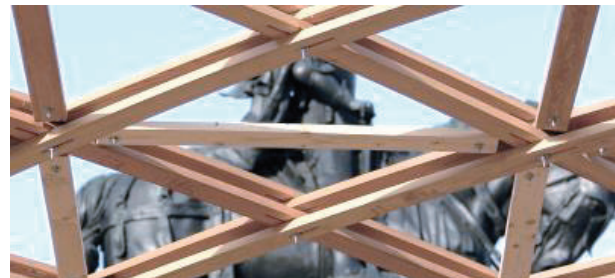
Figure 17- Locking detail of the ZA Pavilion 10
