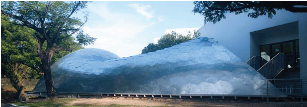
Figure 10- Sutd Library Pavilion 9
