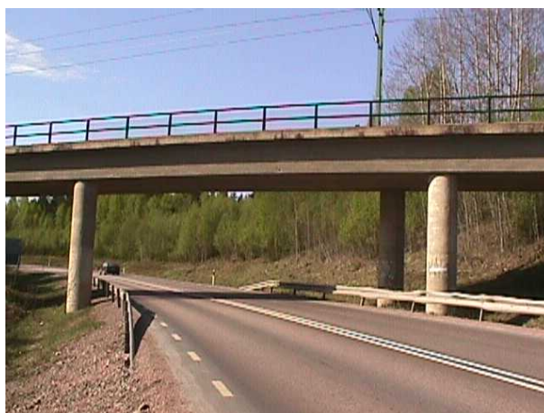
Figure 8.1: 'Brunna Bridge' - photo.
