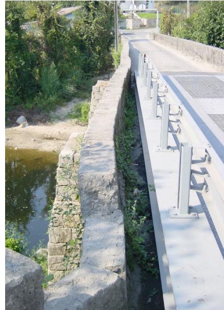
b) Out-of-plane deflection of the spandrel wall.
