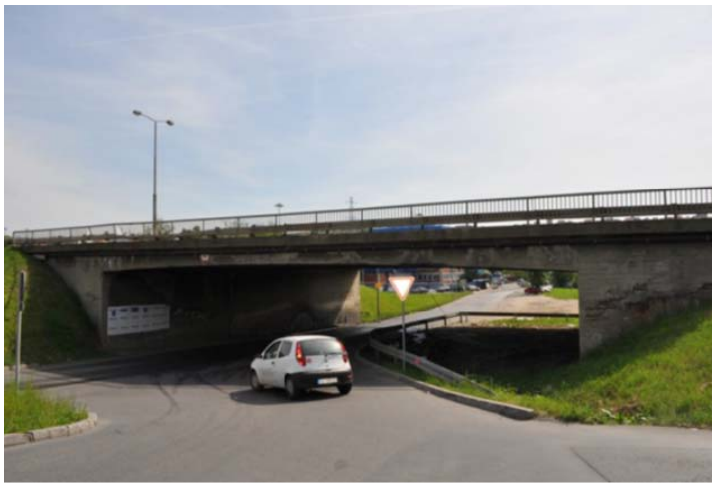
Figure 10. Example: Reinforced concrete frame bridge
