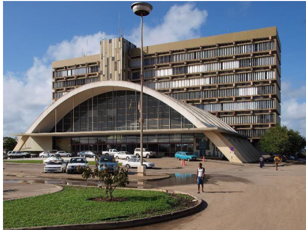
Fig. 10 - Beira Central Station, entrance hall and administration block (Elisiário Miranda, 2009)
