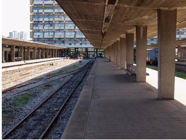
Fig. 12 - Beira Central Station, platforms area and administration block (Elisiário Miranda, 2009)
