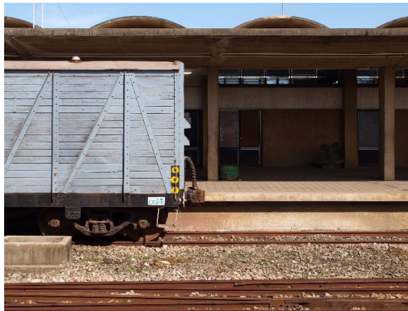
Fig. 14 - Beira Central Station, command building in platforms area (Elisiário Miranda, 2009)
