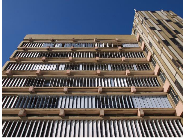
Fig. 13 - Beira Central Station, Administration Block (Elisiário Miranda, 2009)
