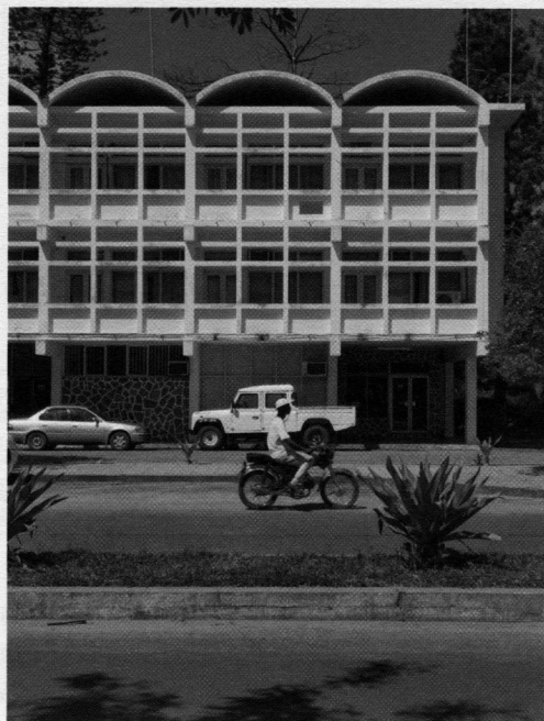
Northeast façade, Elisiário Miranda, 2009
