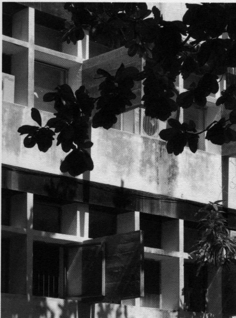
Brise-soleil on the North façade of body II, EWV, Elisiário Miranda, 2010
