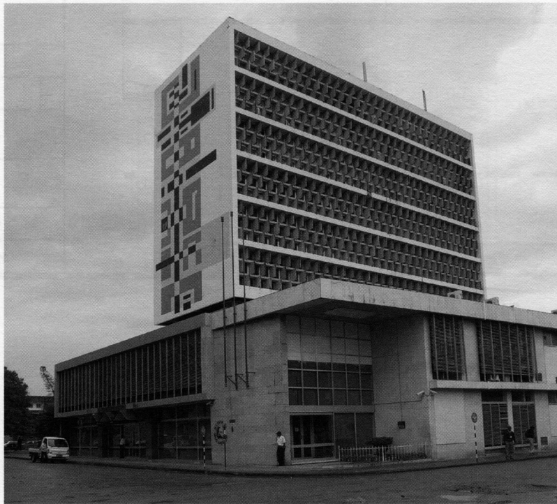
BNU Branch Office in Quelimane, exterior with tile panel by João Aires, EWW, Elisiário Miranda, 2010
