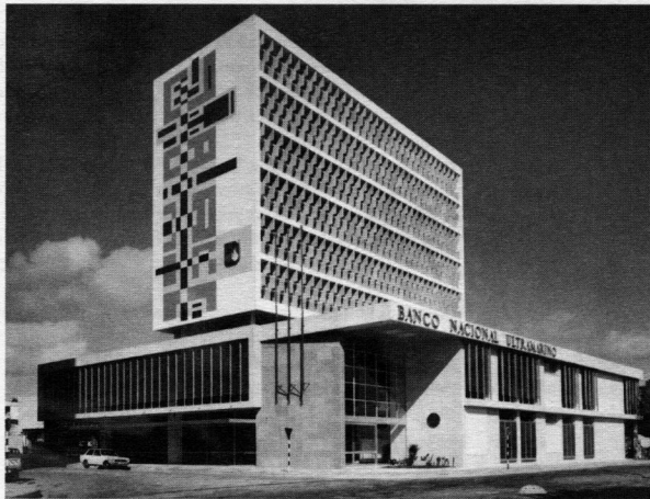
BNU Branch Office in Quelimane, exterior with tile panel by João Aires, Lusitana, undated, AHCGD, Elisiário Miranda, 2010
