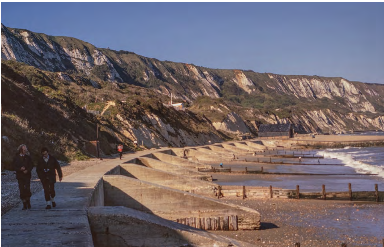
Photo 6.4 Hard engineering with a sea wall to halt cliff erosion and groynes to capture sand might be necessary in places, but alternative soft engineering approaches should be tried first. Folkestone, England. © Roger Crofts
