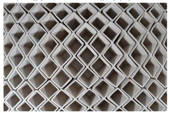
Figure 7. Hive wall - Deficient joins between pieces.
