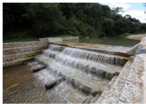
Fig. 6 Dique (Diprotec Geo, 2018)
