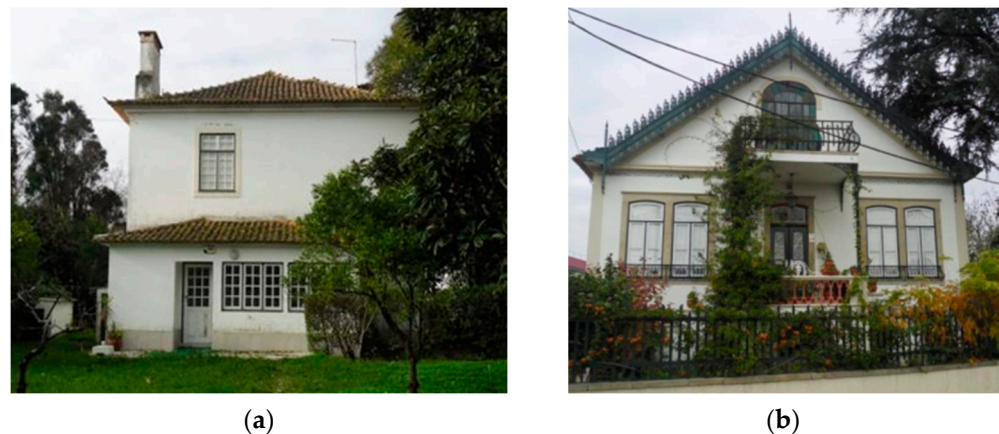
Figure 2. Photographs of the main façades: (a) two-story (Building 2); (b) 2-story plus an attic (Building 3).
