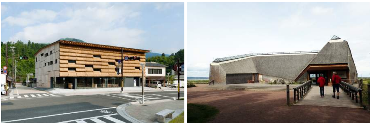
FIGURE 3.6. (left) Community Market Yushara, Japan, completed in 2010 (Architects: Kengo Kuma and Associates) (© Photograph by Takumi Ota [119]); (right) Tåkern visitor centre, Sweden, completed in 2012 (Architects: Wingårdhs) (Photograph by Anna Fuster [120]). The lake 's reeds were used to clad the building.
