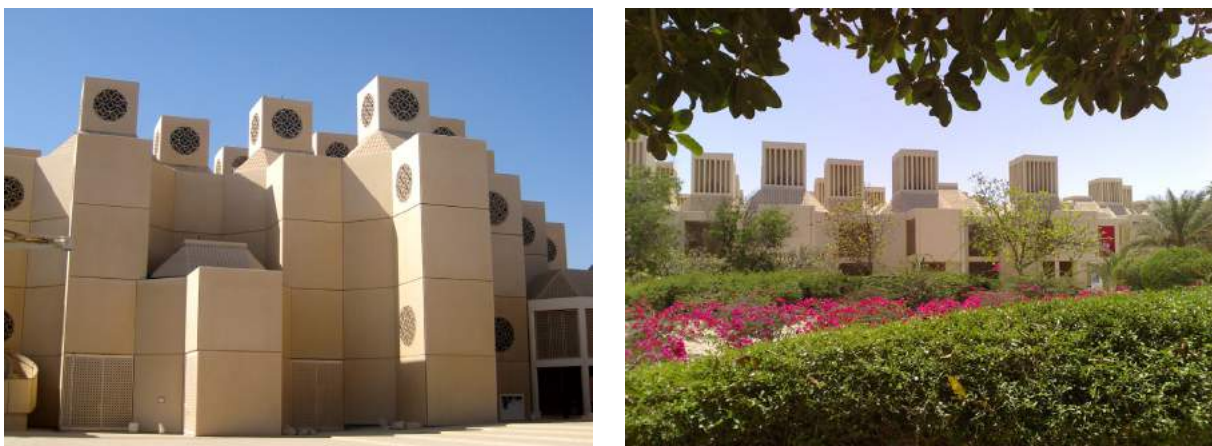
FIGURE 2.3. Wind catchers of the Qatar University building, completed in 1985 (Arch. Kamel El Kafrani). Left [50]; Right [51].
