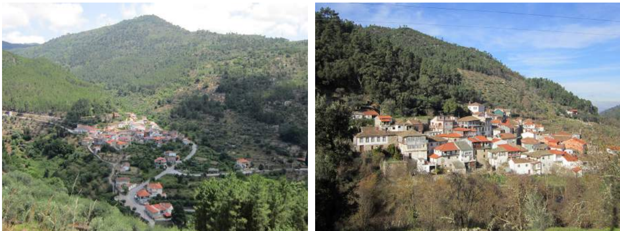
FIGURE 5.26. Granja do Tedo. (left) Upper part, seen from West; (right) Lower part, seen from East.
