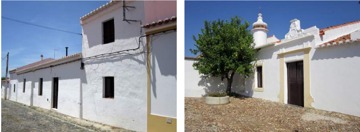
FIGURE 5.47. External views. (left) southeast façade; (right) northwest façade.
