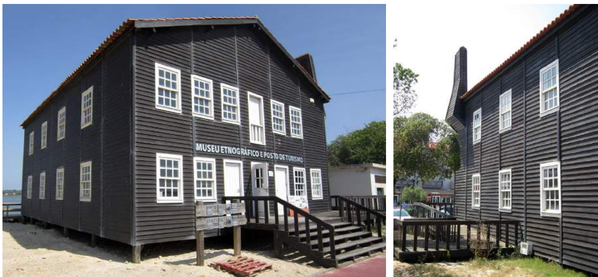
FIGURE 5.10. External views of the case study. (left) north and west façades; (right) south façade.
