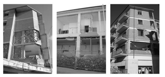
**Figure 1.** Partial and complete out-of-plane collapses of infilled walls during the L'Aquila earthquake (2009), Italy.
