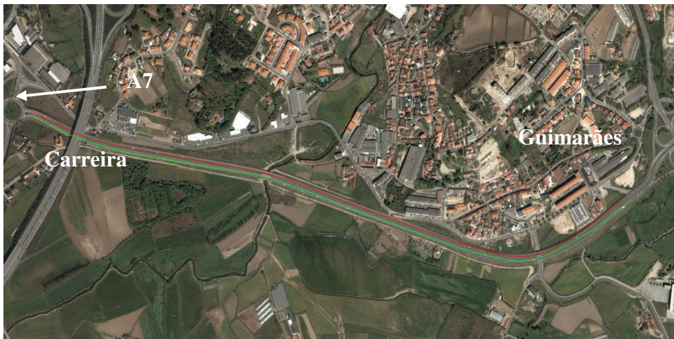
Figure 7. General view of the EN 206 Variant
