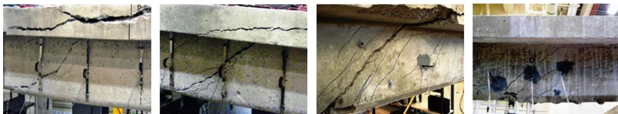
Viga S1- 9d260s
