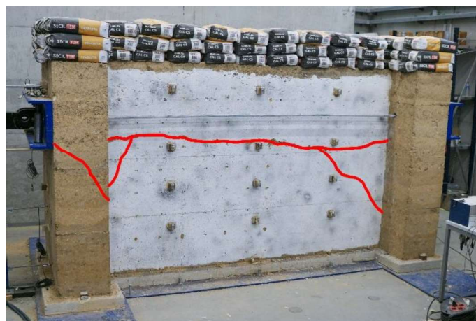
Fig. 3 Cracking pattern of the RE-IP model
